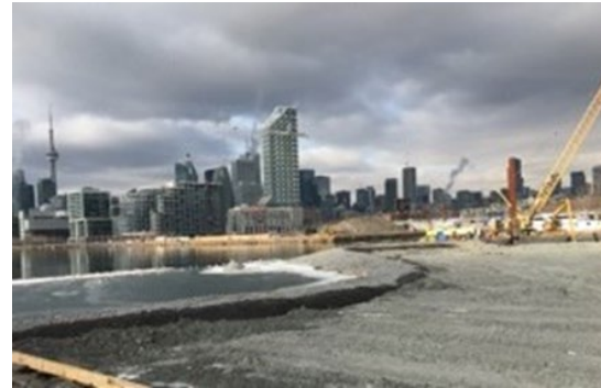
Toronto waterfront, Don River project filling - MECP, Jan. 2019
